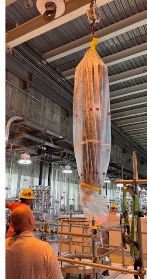
Sleeved Filter Upon Removal
